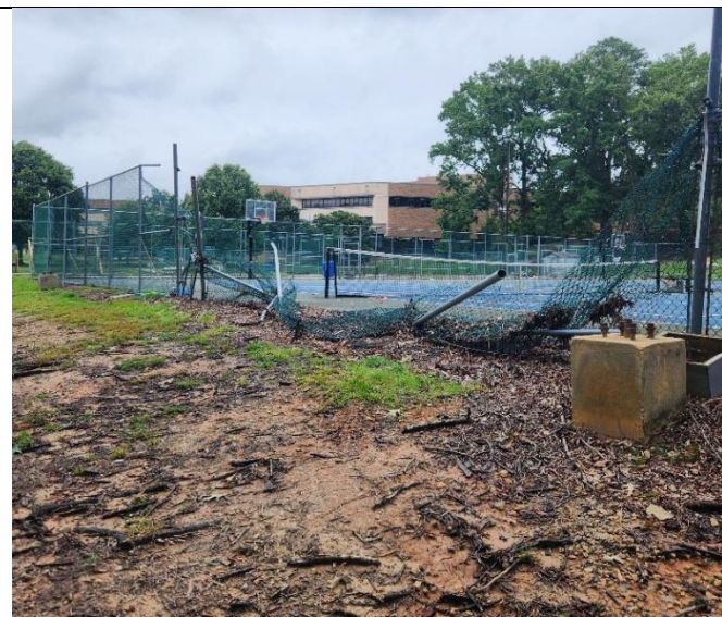
Location 1- Recreational Tennis Court
